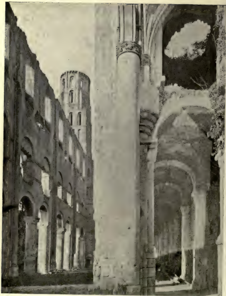
NAVE AND NORTH AISLE, LOOKING WEST Abbey, Jumièges
